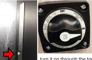
Turn on the battery disconnect and the inverter. If the Dometic system shuts it off,
