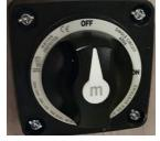
Turn off the battery disconnect and unpress the button on the inverter for ONE minute.
