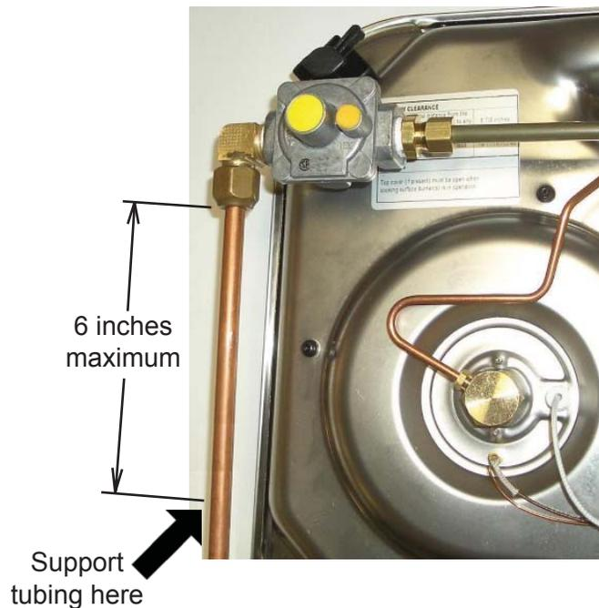
6. **IMPORTANT:** All gas connections must be leak-tested using an RVIA approved test method.
