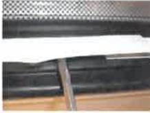
In order to change the sealing rubber, it is necessary to dismantle the windowpane, the clamp holders as well as the opener. Furthermore, the filler profile section must be levered out with the aid of a screwdriver. Loosen rubber at the joint and pull off all around.
