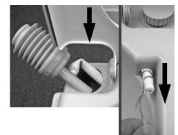
4. Hook wire through holes in hose nozzle and wrap wire around nozzle. Lubricate bulge in nozzle for easier installation in step 6. Pull wire and nozzle end out of small hole in bowl while guiding new bellows pump into position.
