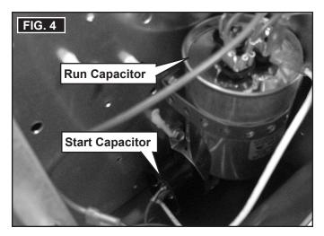
5. Disconnect all wires from run capacitor. See (FIG. 5).
