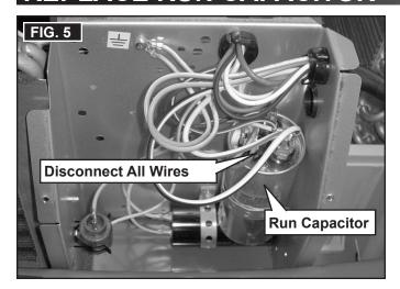
6. Remove and discard run capacitor & capacitor strap (with 2 screws) Save screws for reinstallation later. See (FIG. 6).
