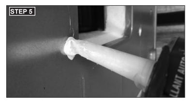
· Cover the four screws with 1021 sealant.
