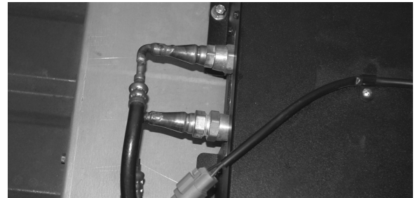
Figure 10: Refrigerant lineset quick-connect fittings
