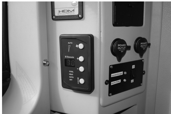
Figure 14: Qt control panel installed
