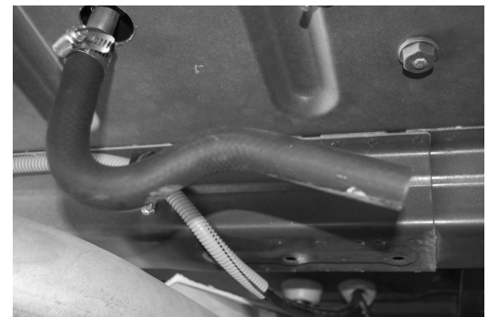
Figure 17: P-trap installed
