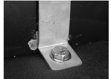
Figure 9: Mounting clip
