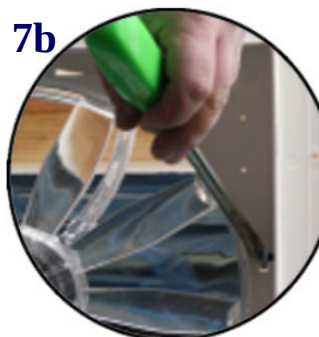
Clean the Knockout
